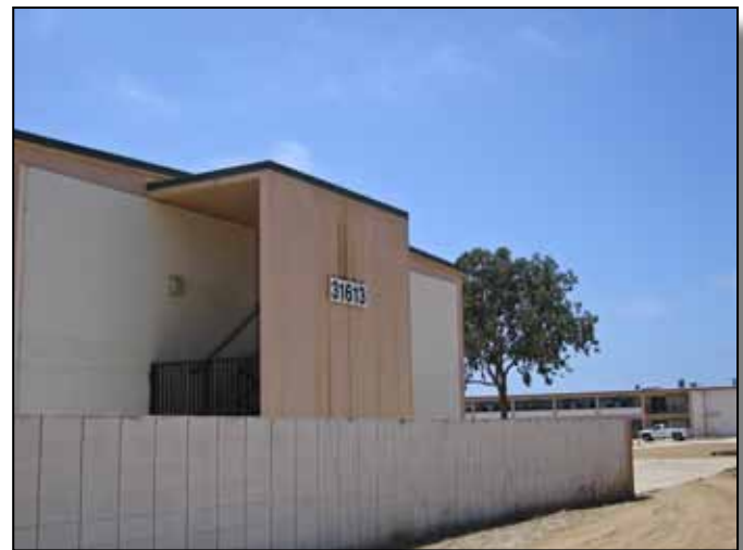
Figure 3.5-28: Lack of downspout gutters has stained Building 31613 in Edson Range (31A) Area.
