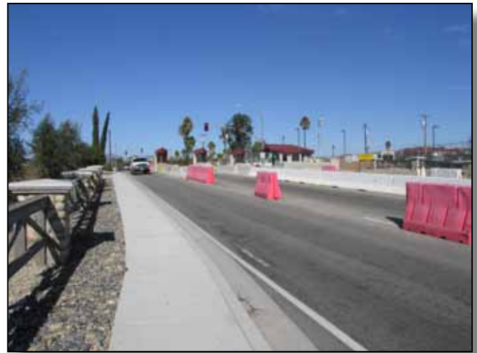
Figure 6.3-3: Clear view of vehicle travel lanes with queuing.
