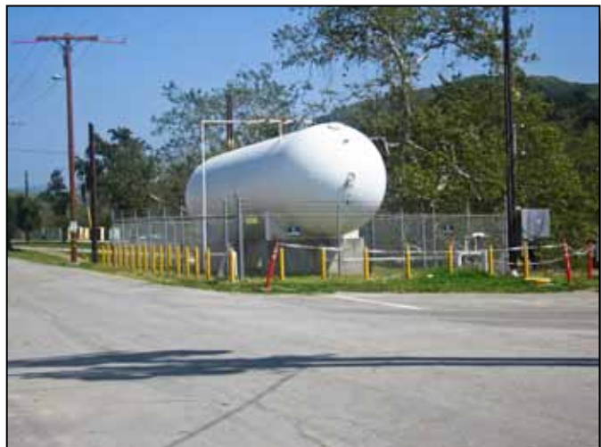
Figure 4.20-11: Above ground storage tanks lack screening.
