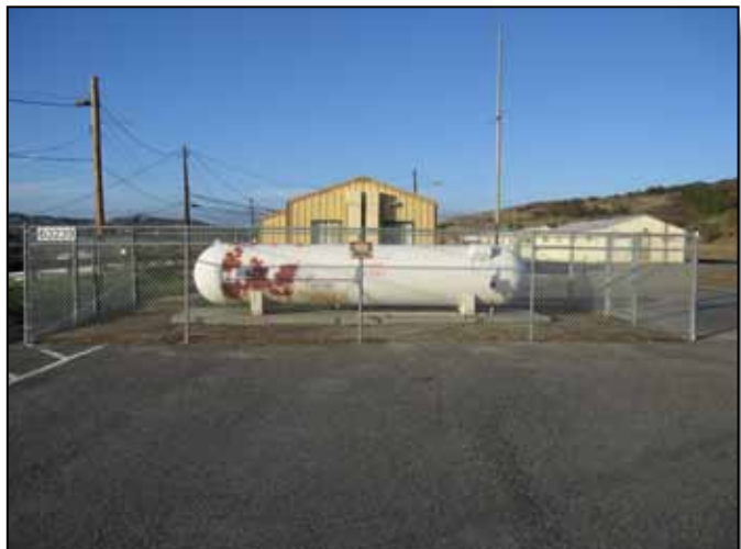
Figure 3.17-5: Chain link fence at AST, still lacks screening.
