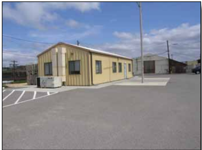
Figure 4.19-5: Temporary building in the administration area.
