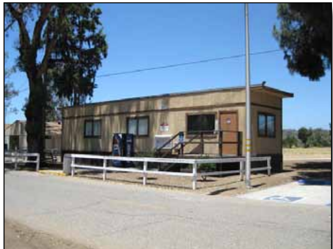
Figure 5.2-10: Office at Lake O'Neill Campground.
