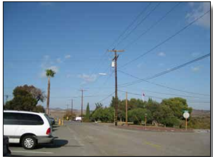
Figure 4.13-12: No separation between the street and parking at the Headquarters building.
