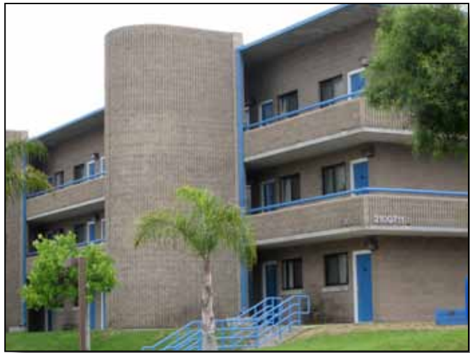
Figure 4.3-5: Older BEQ in need of upgrading.
