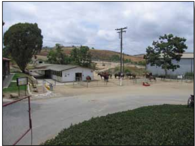
Figure 5.6-2: Building 1515 is an example of appropriate stable character.
