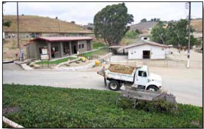
Figure 5.6-5 Variety of architectural styles found throughout the stable area.
