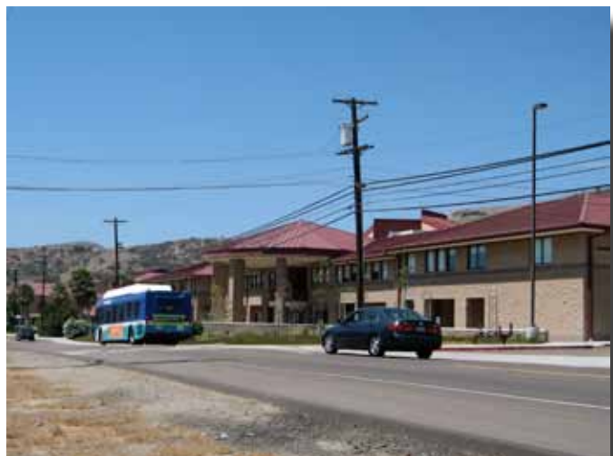
Figure 4.18-4: Newer building sets design precedent for future development.
