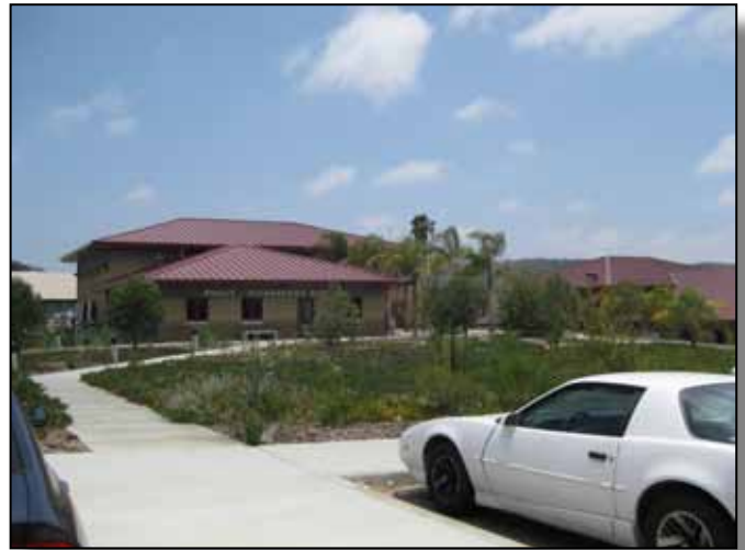
Figure 3.5-7: Building 25118 in Vado del Rio (25) Area is a good example of architecture following BEAP guidelines.
