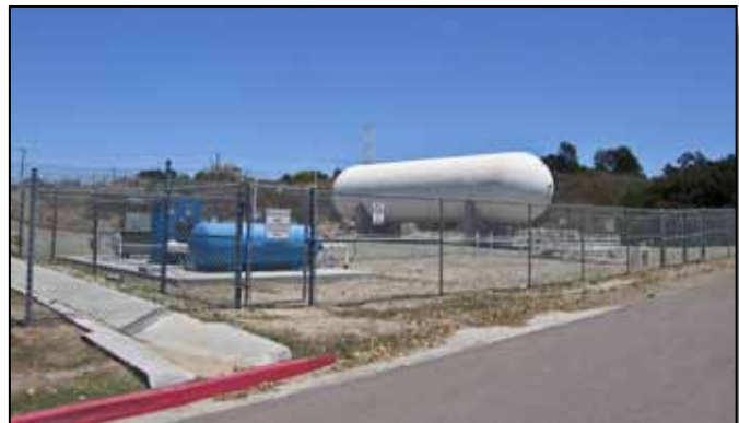
Figure 3.14-2: Exposed propane tank at Naval Hospital (27) Area.
