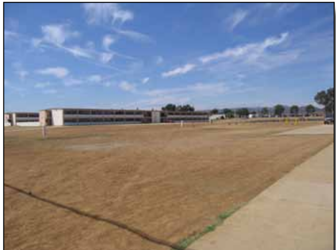
Figure 4.9-6: Extensive areas of dirt at BEQs.
