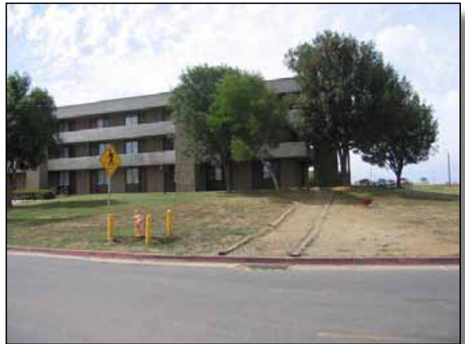
Figure 3.4-2: Lack of permanent pedestrian path at the Las Flores (41) Area.
