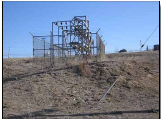
Figure 4.3-8: Substation on the south side of Harbor Road.
