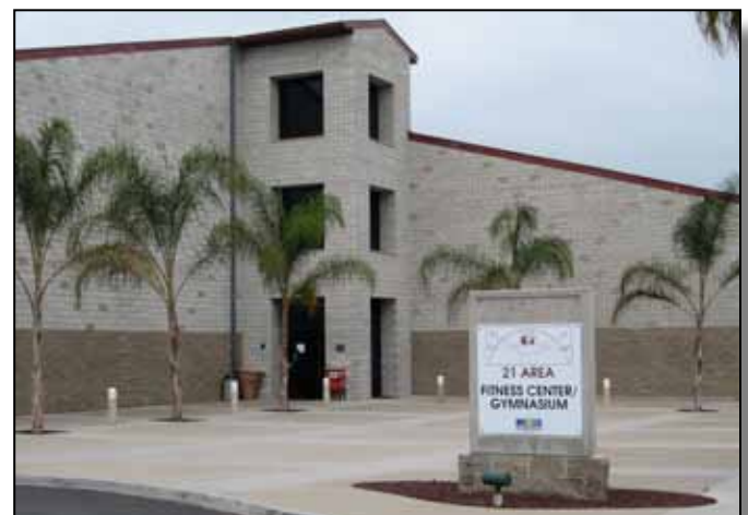
Figure 3.10-20: MCCS Facility Sign in the Del Mar (21) Area.
