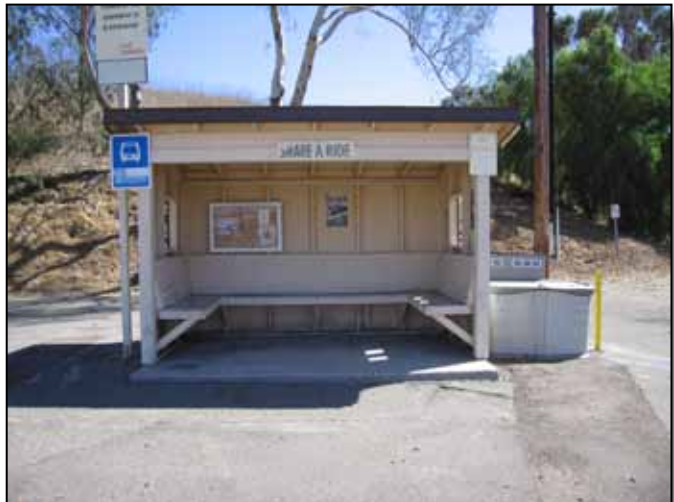
Figure 3.15-1: Existing bus shelter to be replaced.
