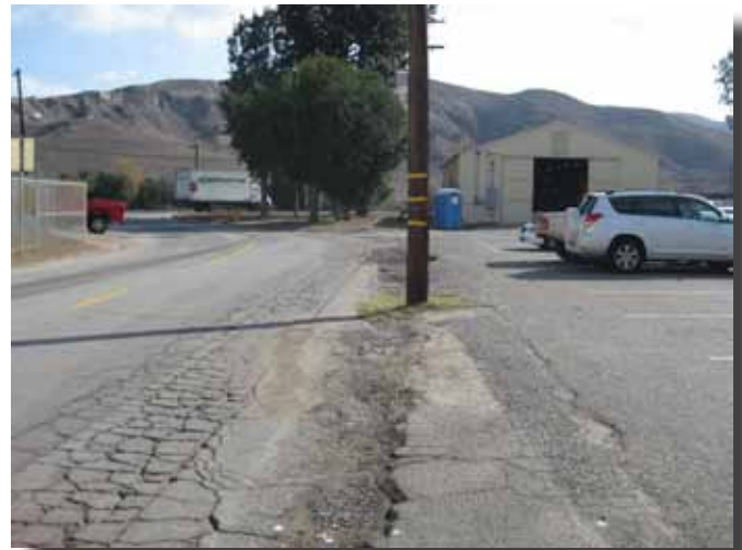
Figure 4.15-11: Lack of separation between streets and parking.
