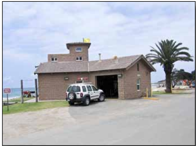
Figure 5.4-5: Lifeguard Station Building.
