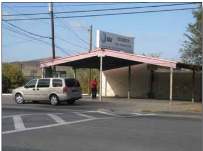
Figure 3.5-6: Abandoned phone center at Horno (53) Area.
