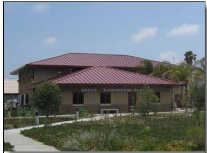
Figure 4.6-8: Building 25118 is a good example of architecture following BEAP guidelines.
