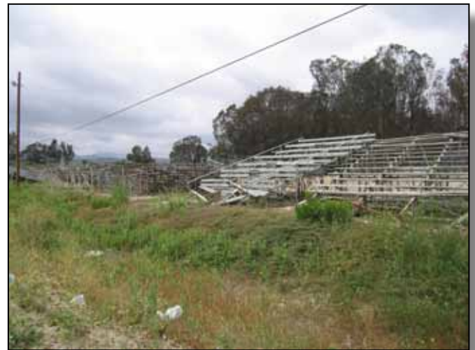
Figure 4.7-6: Unscreened storage of broken bleachers.
