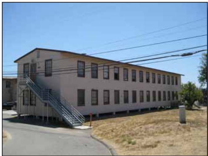
Figure 3.5-5: Building 1244 in the HQ Area.
