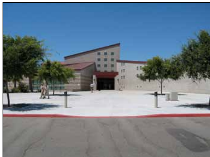
Figure 3.2-1: Paige Fieldhouse - example of good design on Base.
