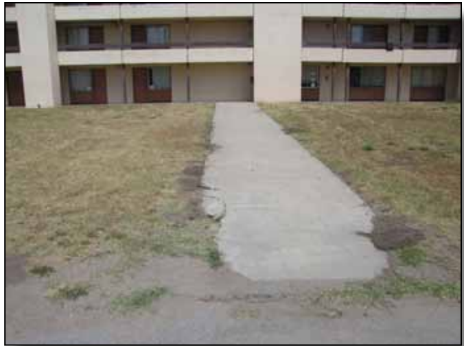
Figure 4.17-5: Sidewalk between parade grounds and Building 53323.
