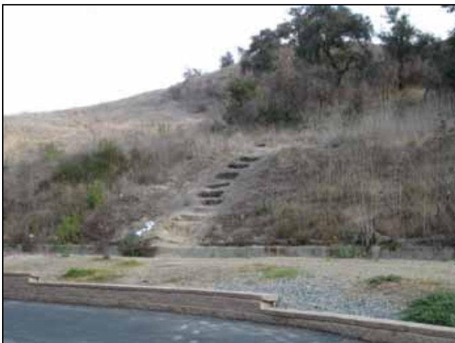
Figure 4.17-17: Existing stairs are unsafe and need replacement.
