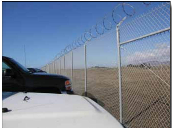
Figure 4.11-7: Area is surrounded by a secure perimeter chainlink fence.
