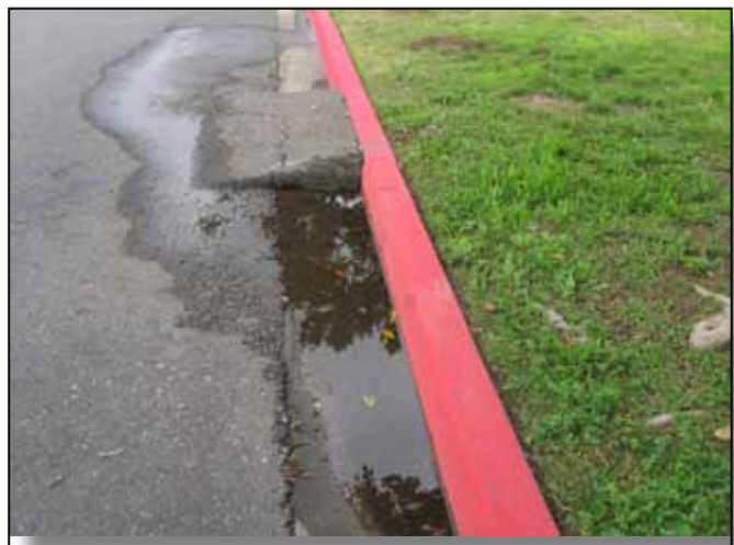
Figure 4.8-6: Irrigation runoff caused by poor monitoring of irrigation systems.
