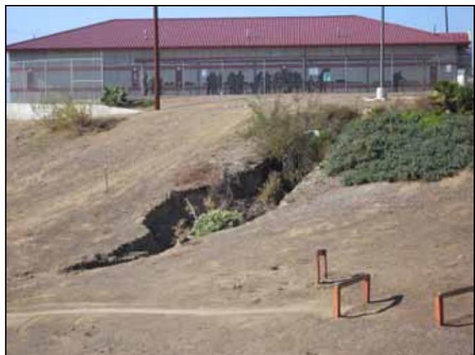
Figure 4.3-7: Eroded slopes on the north side of Harbor Road. Also note the above grade utility lines.
