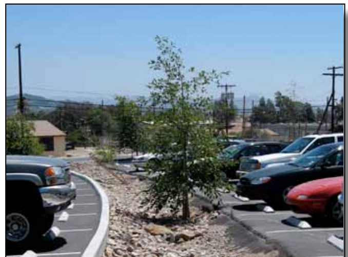
Figure 2.3-4: Example of a drainage swale in a parking lot on Base. Water is filtered through cobble before going into a storm drain or other suitable dispersion method.
