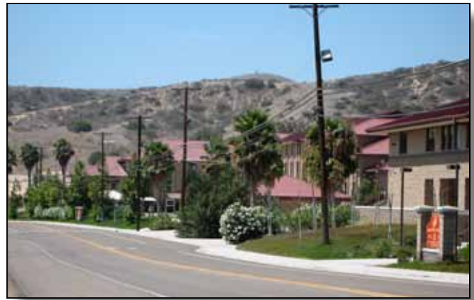
Figure 3.14-4: Overhead power lines cause visual clutter throughout the Base.
