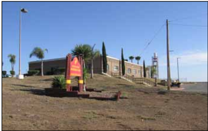
Figure 4.12-6: Existing building in Mass (32) Area.
