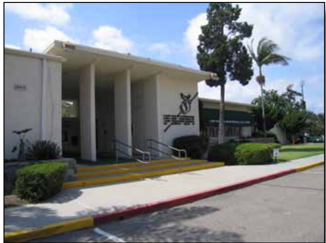
Figure 5.5-2: Main entry to clubhouse Building 18415.
