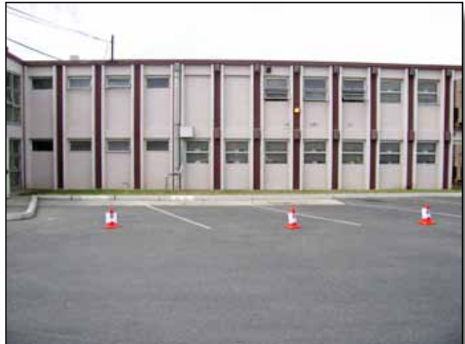
Figure 4.14-5: Example of non-conforming parking adjacent to building in the Las Flores (41) Area.
