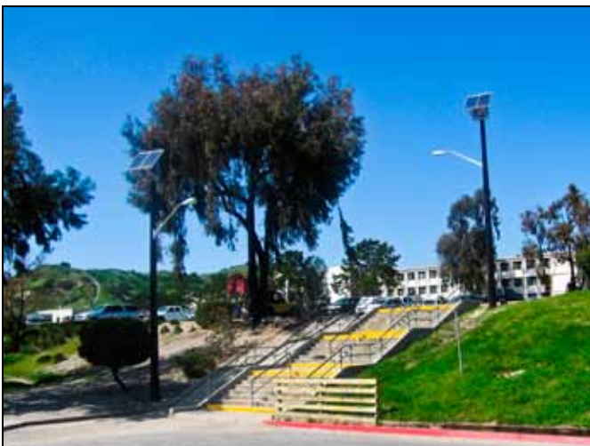
Figure 4.16-15: Existing lighting at stairway leading to parking lot.
