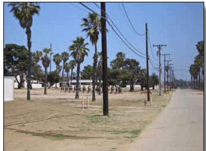
Figure 4.9-14: Above ground utilities create visual clutter.
