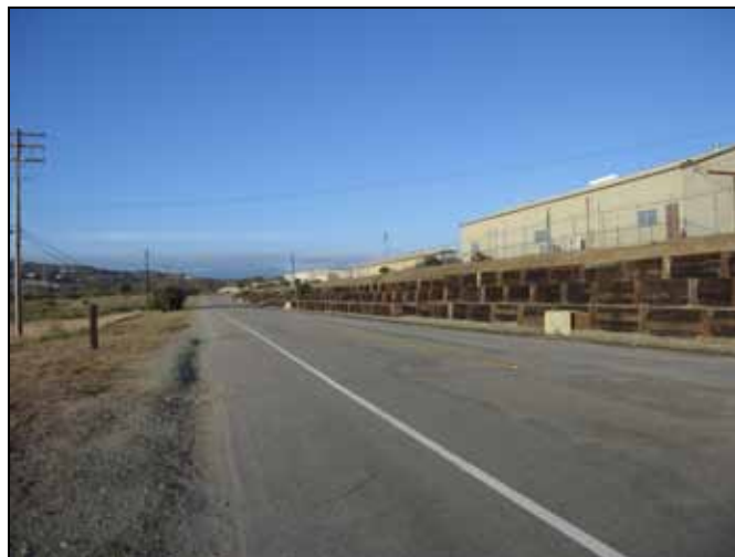
Figure 4.19-2: Cristianitos Road is wide enough for a bicycle and/or pedestrian path.
