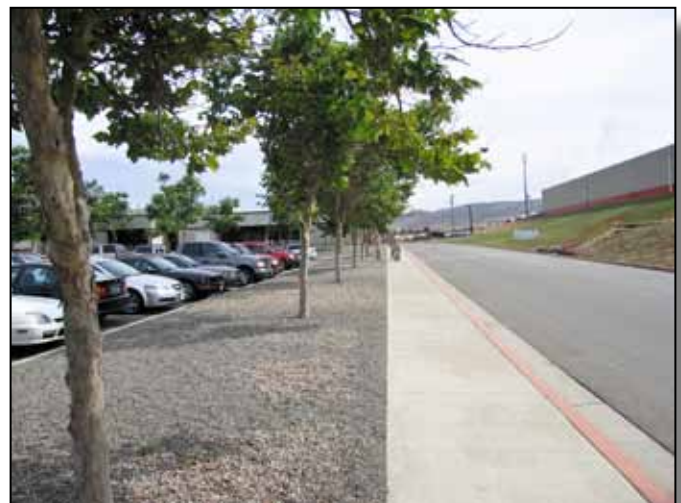
Figure 3.7-6: Pedestrian sidewalk, contiguous with curb, in Las Flores (41) Area.
