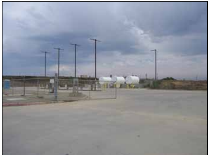
Figure 3.17-4: Unobstructed access to AST.
