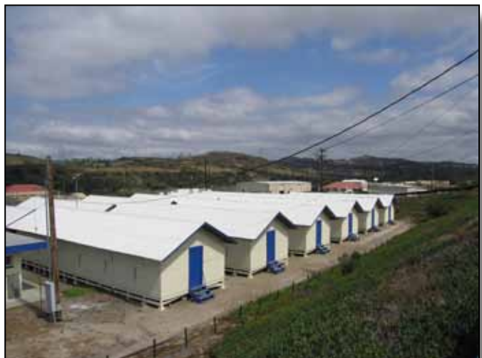
Figure 4.19-6: Existing temporary buildings at Cristianitos.
