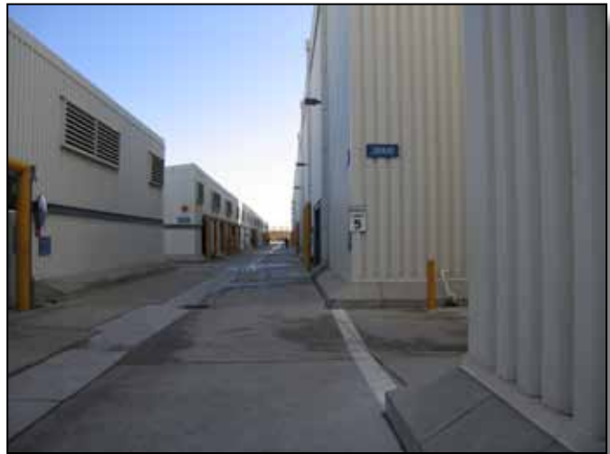
Figure 4.11-13: Existing pre-engineered metal building structures.
