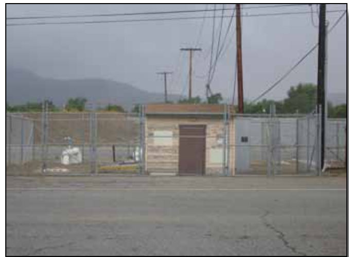
Figure 3.5-34: Use of chainlink fence alone for screening is unacceptable.
