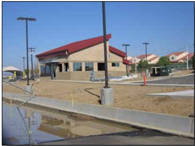
Figure 3.10-7: Oceanside Gate during construction.
