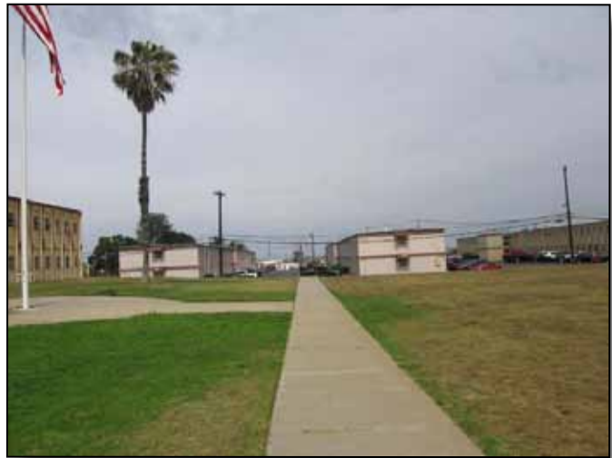
Figure 4.14-4: Views west toward Buildings 41344 and 41346 encompass extensive use of turf.
