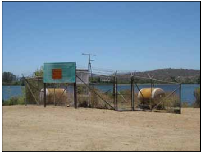
Figure 5.2-18: Unscreened utilities in the day use area.
