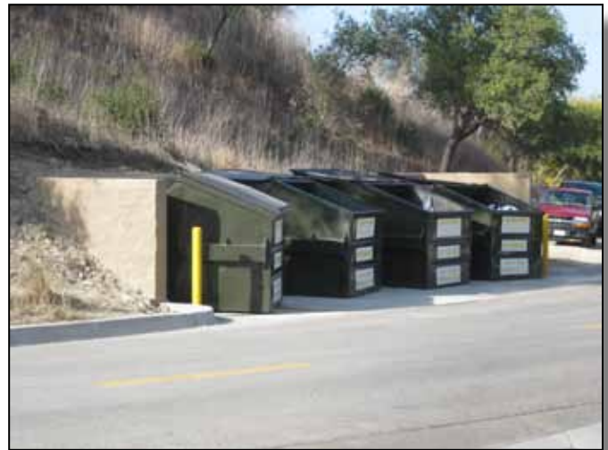
Figure 3.16-4: Enclosure wall around dumpsters along a service road.
