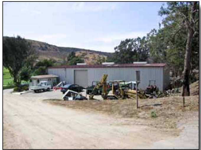
Figure 5.5-8: Existing dirt road to maintenance buildings.
