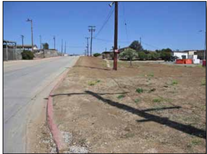
Figure 3.9-2: No sidewalks along Nelson Road to Building 41404 in Las Flores (41) Area.
