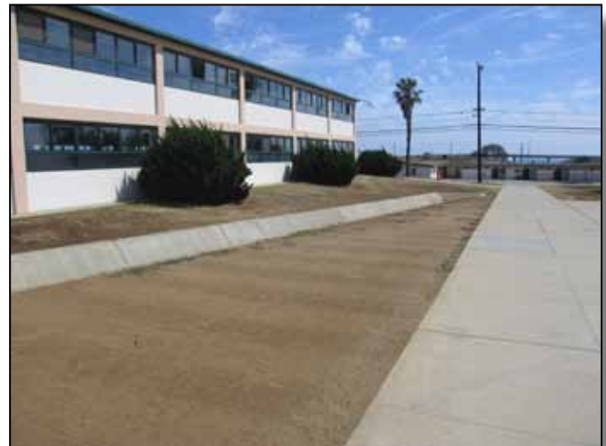
Figure 4.9-9: Existing concrete buildings at Edson Range (31A) Area.
