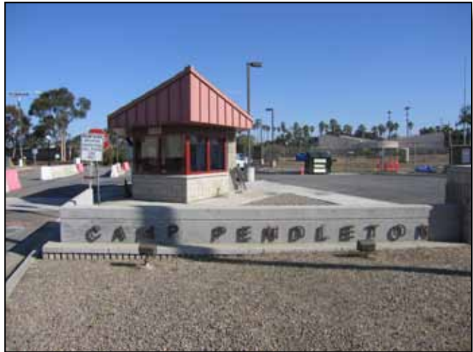
Figure 6.7-1: Del Mar Gate and guardhouse.
