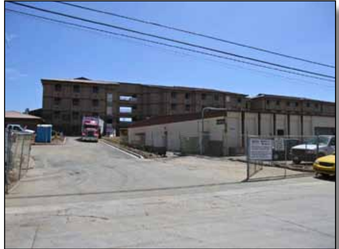
Figure 10.1-1: BEQ under construction.
