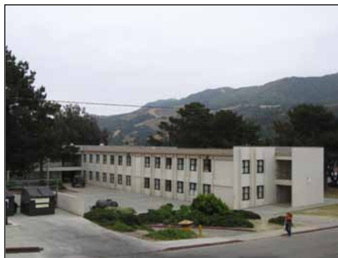
Figure 4.16-3: Building 520442 with hills in the background.
