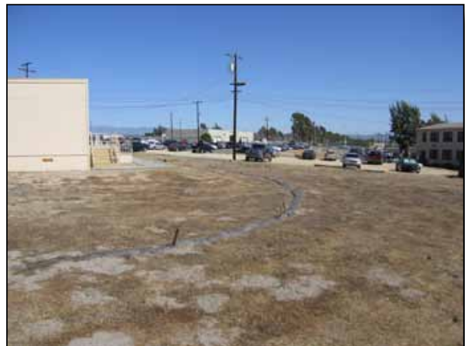
Figure 4.2-21: Above ground utilities cause visual clutter and should be avoided.
