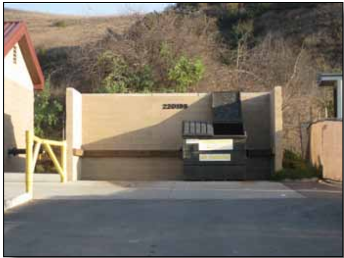
Figure 3.16-6: Wooden rails are not allowed within enclosure.
