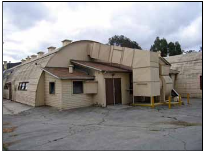
Figure 4.20-5: WWII Quonset huts beyond their service life.
