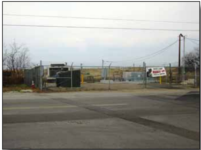
Figure 4.14-15: Unscreened utilities in Las Flores (41) Area.
