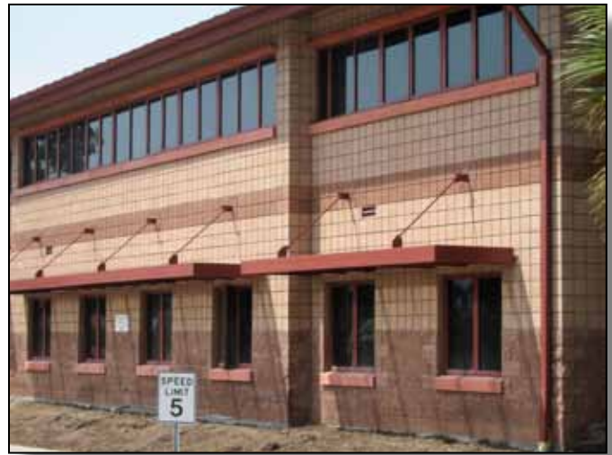
Figure 4.5-7: Newer building in the Pico (24) Area.
