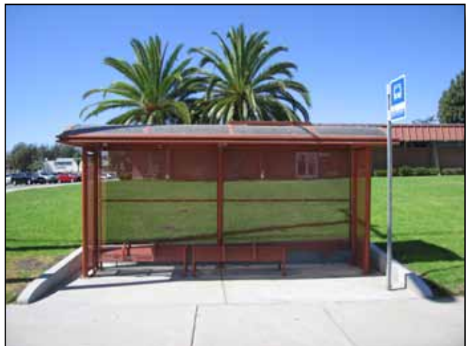
Figure 3.15-2: Approved Primary Bus Shelter on Base.
