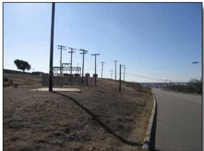
Figure 4.3-9: Above ground utilities create visual clutter.
