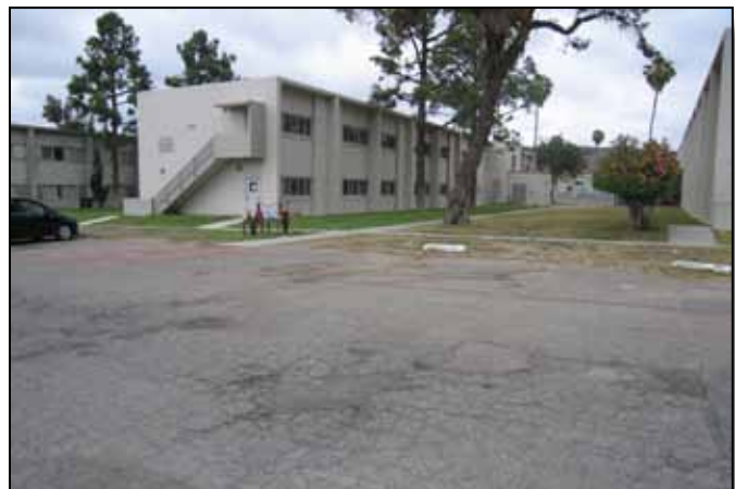
Figure 4.4-18: Parking lot without curbs or landscaping.
