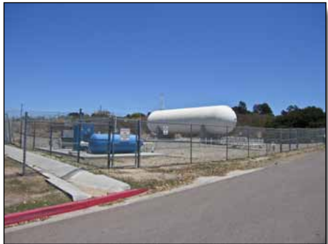
Figure 4.8-10: Visually exposed above ground tank with chain link fence.
