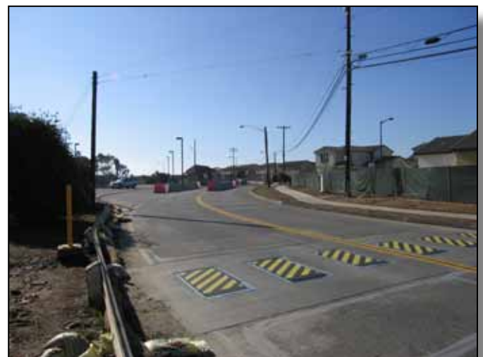
Figure 6.7-3: Overhead utility lines add to visual clutter.
