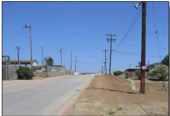
Figure 4.14-16: Overhead utilities in Las Flores (41) Area create visual clutter.
