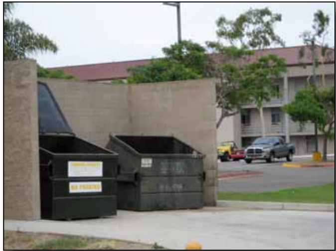
Figure 3.16-1: Trash enclosure in the Del Mar (21) Area.
