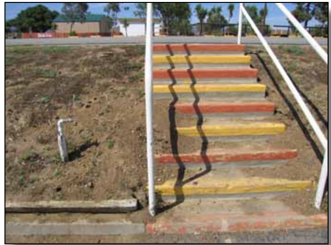
Figure 4.9-8: Typical stair railing with peeling paint.
