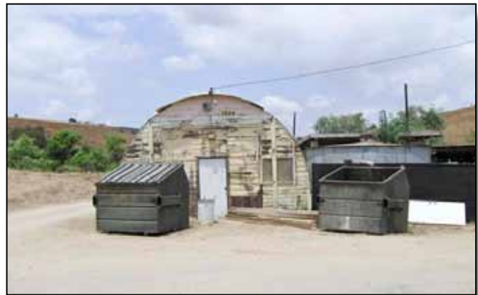
Figure 5.6-6: Existing buildings at stables in need of rehabilitation.
