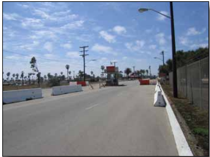
Figure 4.9-5: Entry guard house for Edson Range (31A) Area.
