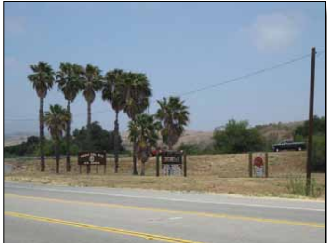
Figure 4.6-3: Vado Del Rio (25) Area identification signs.
