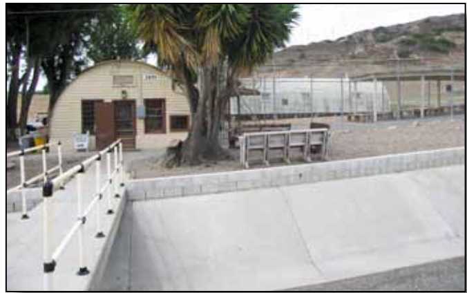
Figure 3.14-1: Open drainage swale in Pico (24) Area.
