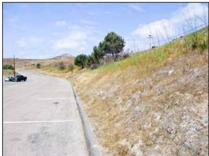
Figure 5.5-7: Slope at edge of parking lot in need of erosion control planting.
