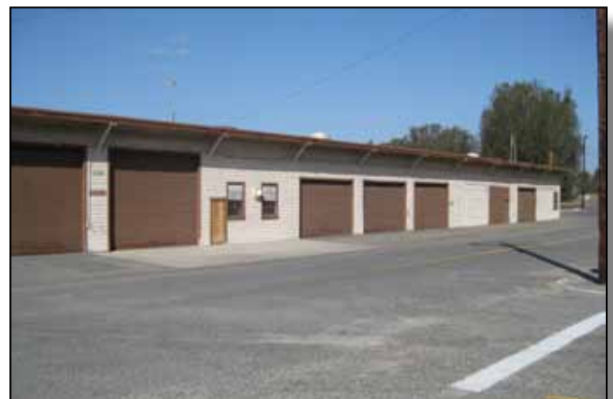
Figure 9.13-5: Access from parking lot to 1942 period building near the Museum.
