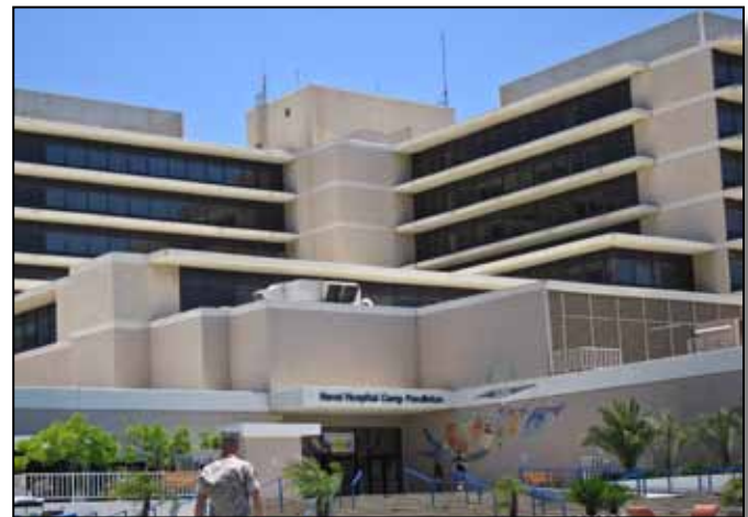
Figure 3.13-2: Exposed roof equipment at Naval Hospital (27) Area.
