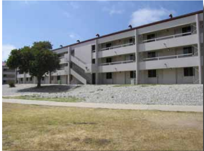
Figure 4.18-2: Looking north to BEQ Building 62430.
