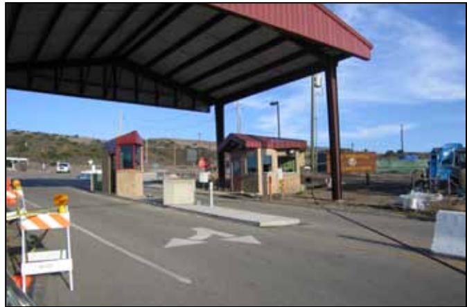
Figure 6.6-2: Canopy over entrance.
