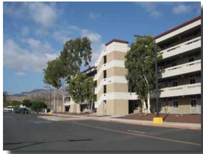
Figure 4.15-6: Newer BEQ using Base approved building colors and materials.
