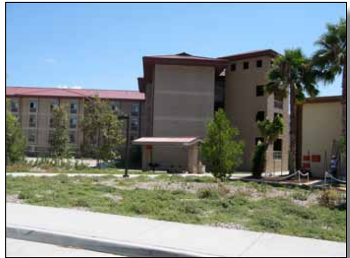
Figure 4.18-8: Newer BEQ is a good example of BEAP approved architecture and enclosed stairways.
