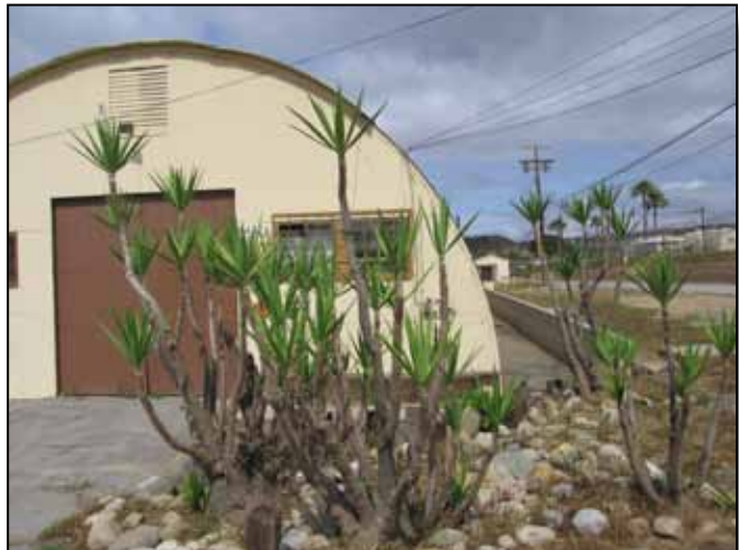
Figure 4.20-3: Use of cobble and low water use plants at Quonset Huts.
