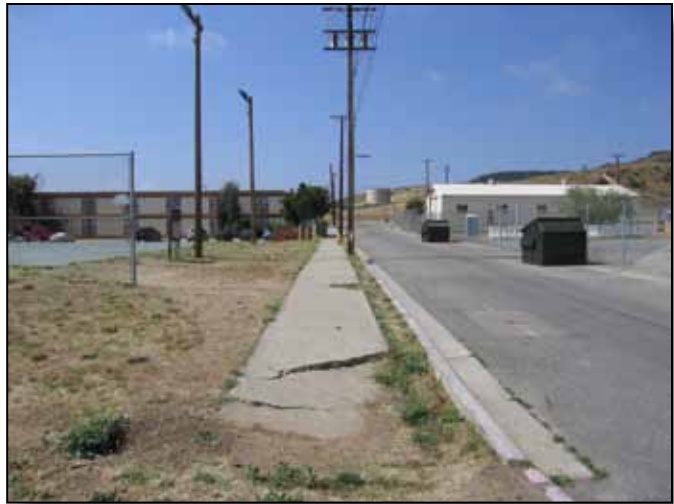
Figure 4.18-5: Broken sidewalk is in need of replacement.
