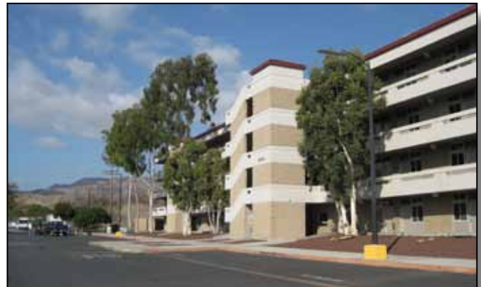
Figure 3.5-22: Enclosed stairwell at building 43700 in Las Pulgas (43) Area-example of preferred design.
