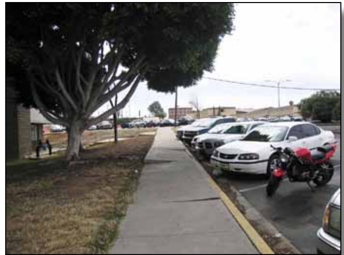
Figure 4.14-6: Example of inappropriate tree choice (roots heaving sidewalk) in the Las Flores (41) Area.
