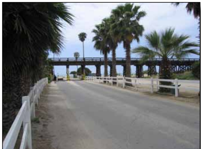
Figure 5.4-4: Entry road prior to beach use.
