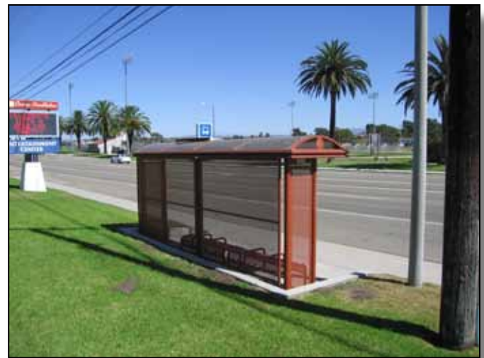
Figure 3.15-3: Rear view of Approved Primary Bus Shelter.
