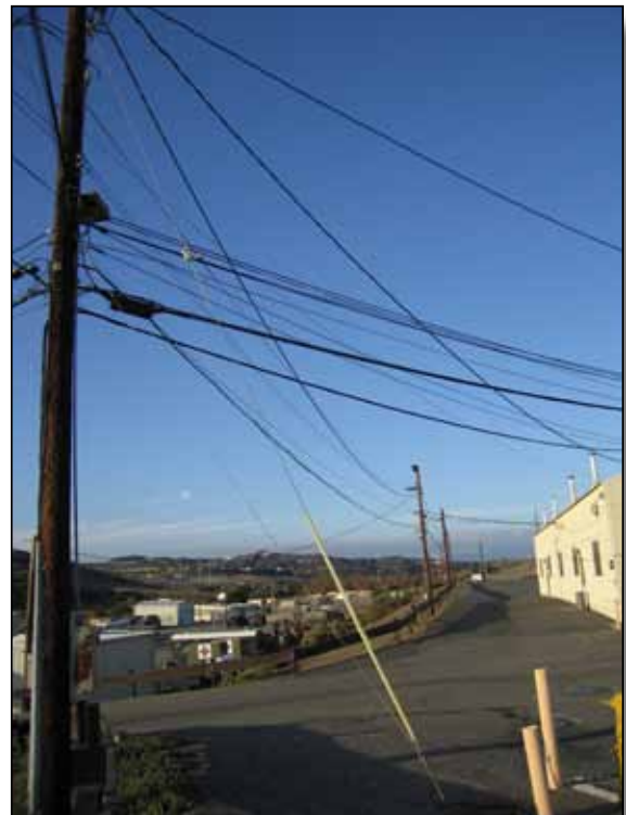
Figure 4.19-13: Above ground utilities cause visual clutter.
