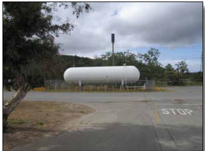
Figure 3.17-2: Bollards surrounding AST in Talega (64) Area.
