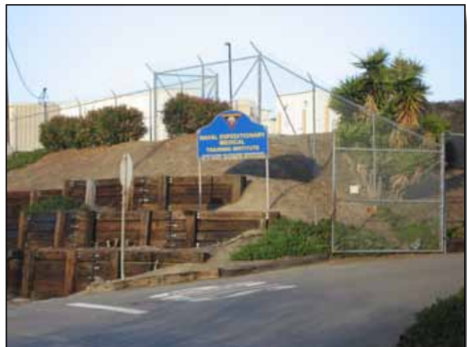
Figure 4.19-10: Existing identification signage.
