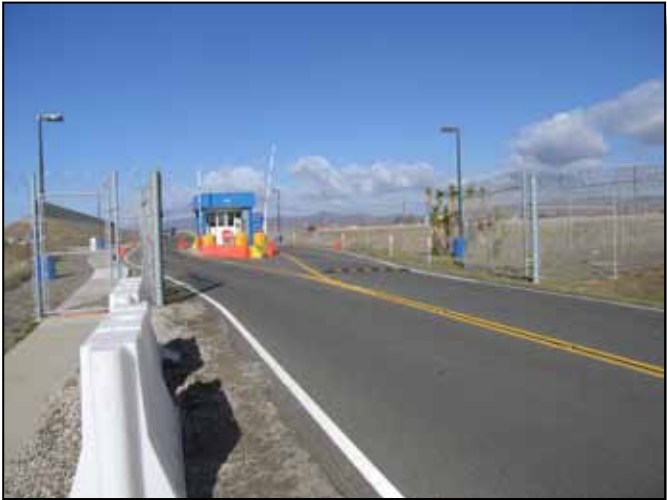
Figure 4.11-12: Area entry lacks vehicle deterrent features.
