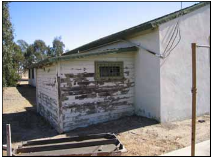
Figure 3.5-4: Older building in state of disrepair.
