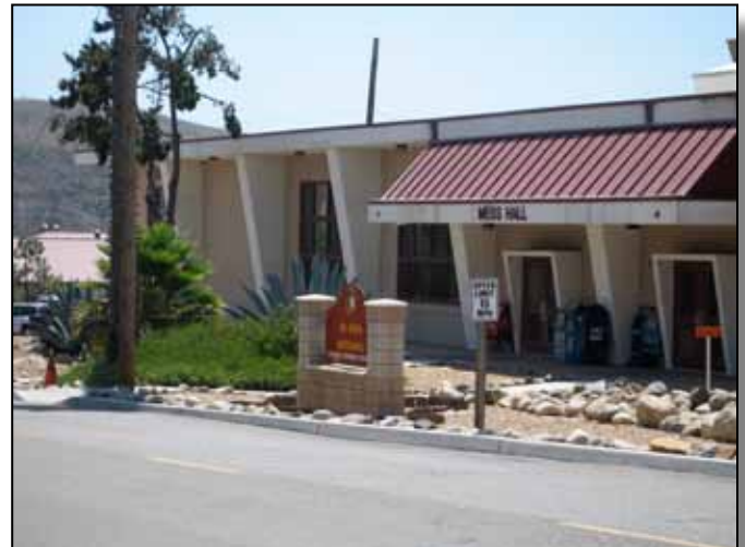
Figure 4.18-9: Older building which conforms to Basewide color scheme.
