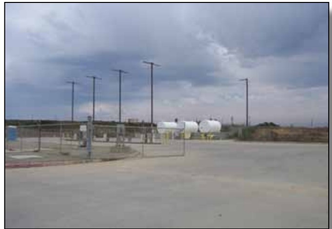
Figure 3.13-1: Above ground storage tanks at MASS (32) Area.
