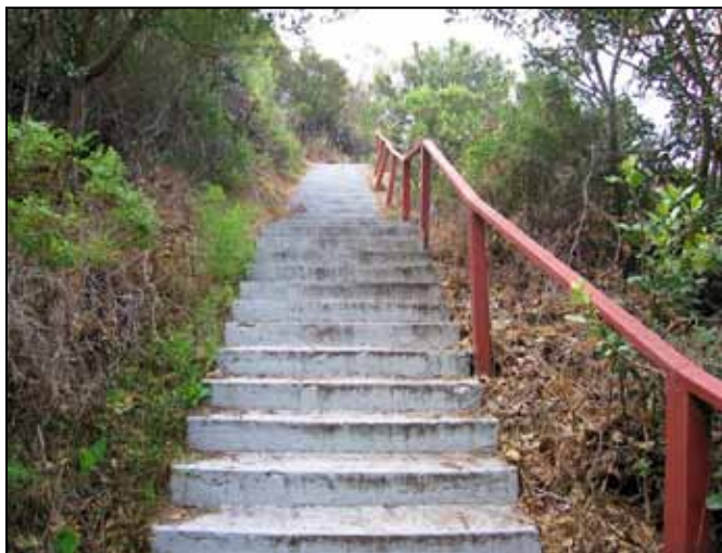
Figure 9.17-4: Stairs leading to site are in disrepair.
