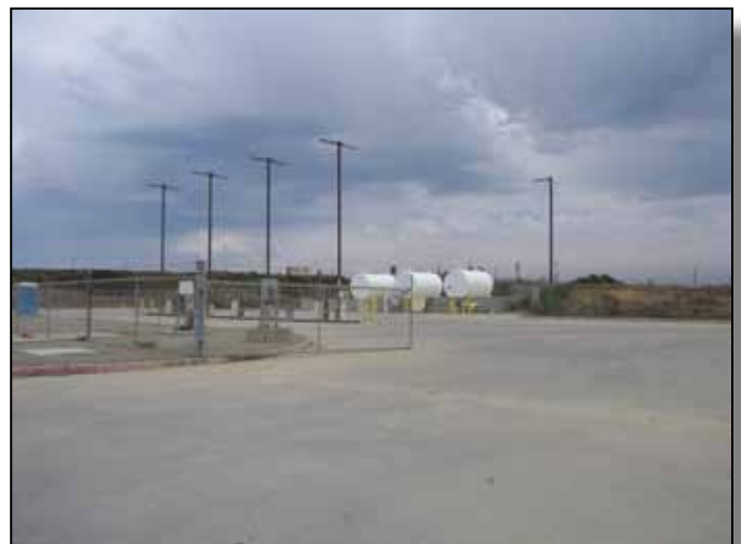
Figure 4.12-13: Screen above ground storage tanks.
