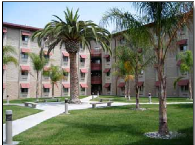
Figure 2.3-3: Newly constructed BEQ adhering to AT/FP design criteria.
