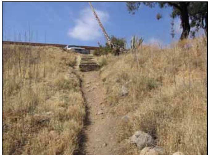
Figure 4.18-6: Narrow stairs and eroded slopes leading to BEQ Building 62431.
