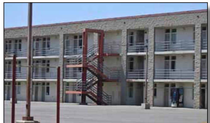
Figure 3.5-23: Open stairwell at BEQ. Example of poor design and non-conforming BEAP design.
