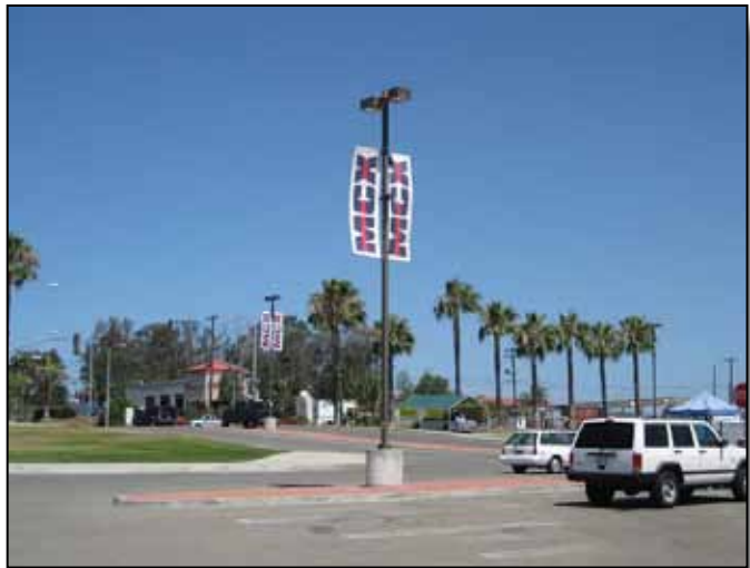
Figure 4.2-20: Example of appropriate light fixture at MCX parking lot.
