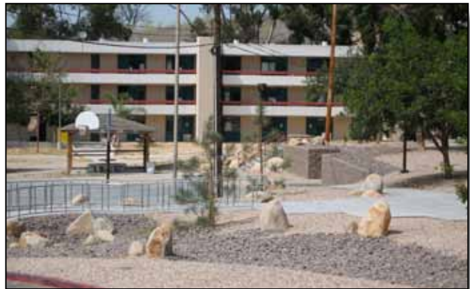
Figure 4.5-9: Cobble and gravel used as permeable ground cover.
