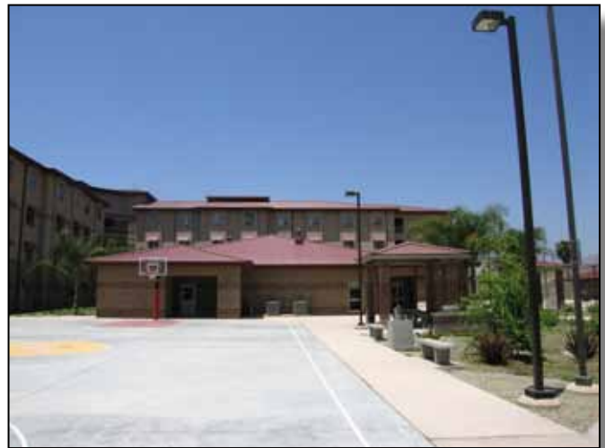
Figure 4.17-3: Newer BEQ Building 53574.
