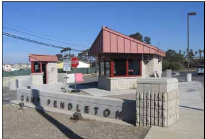
Figure 6.7-2: Sentry booth and guardhouse.
