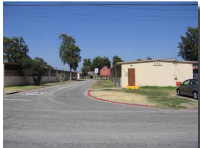
Figure 4.15-7: Older one story buildings throughout the Las Pulgas (43) Area.
