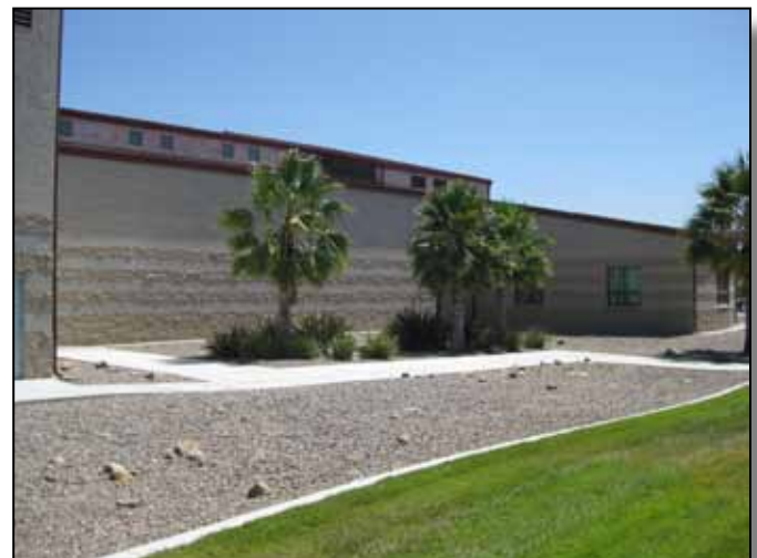
Figure 3.5-29: Precision block with accent banding of splitface block.
