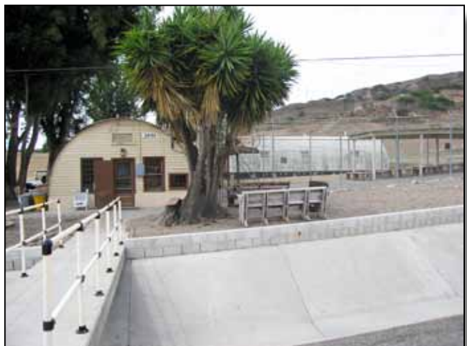
Figure 4.5-6: Concrete flood channels near Building 24111.
