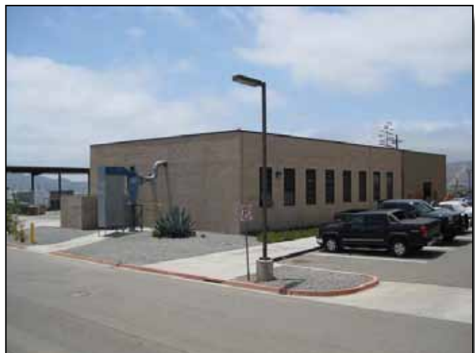
Figure 4.6-4: Example of inappropriate color for exterior building equipment.
