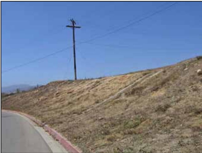
Figure 2.3-2: Example of soil erosion on Base, due to lack of vegetation on slopes.
