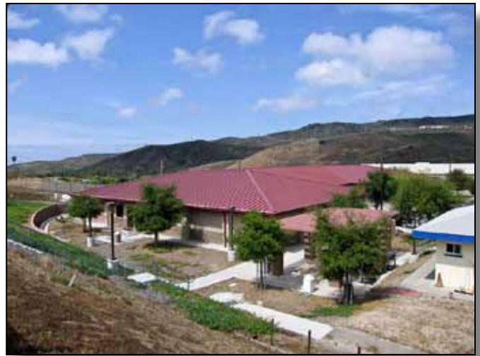
Figure 3.4-1: Older and newer buildings at Cristianitos (63) Area.
