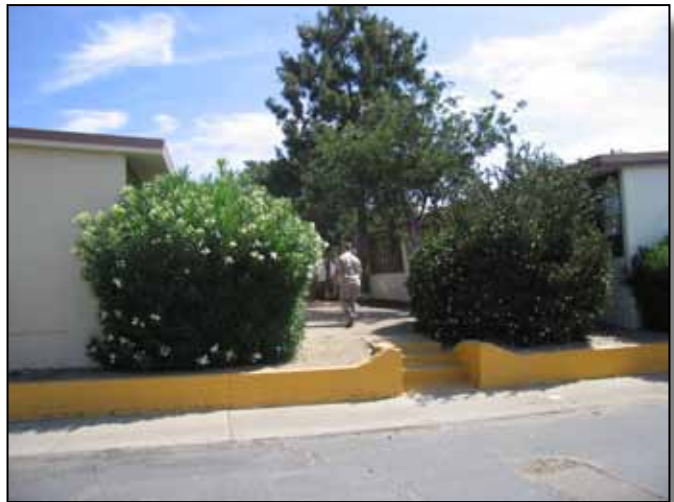
Figure 4.13-5: Pedestrian walk and stairs in need of upgrading at Building 33326.
