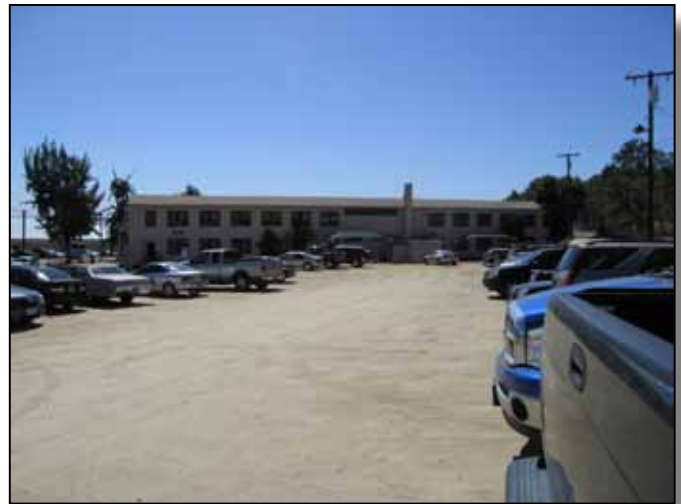
Figure 3.8-1: Overflow parking at Building 1331 in the HQ Area.
