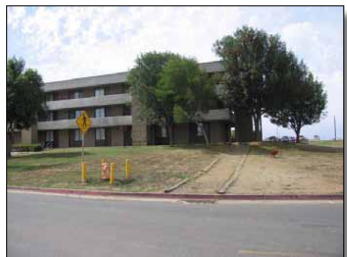
Figure 4.14-14: Substandard path to Building 41303.
