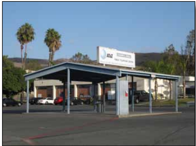
Figure 3.12-9: Typical telephone Vendor shelter no longer in use
