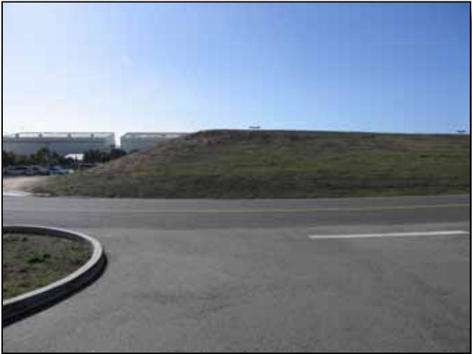
Figure 4.11-9: Large berms are subject to erosion.
