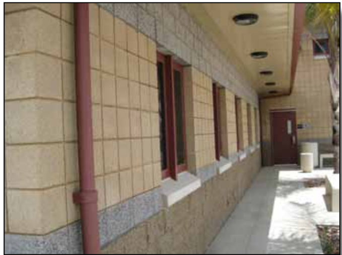
Figure 3.5-32: Precast concrete window sill in Vado del Rio (25) area.
