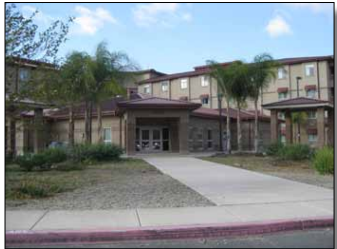
Figure 3.5-2: Newer BEQ, Building 530642, in Horno (53) Area.
