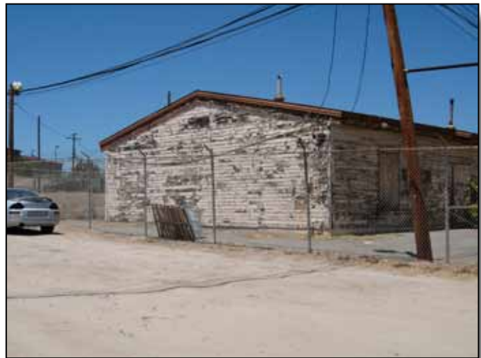
Figure 4.2-6: Older building in need of repair or replacement.
