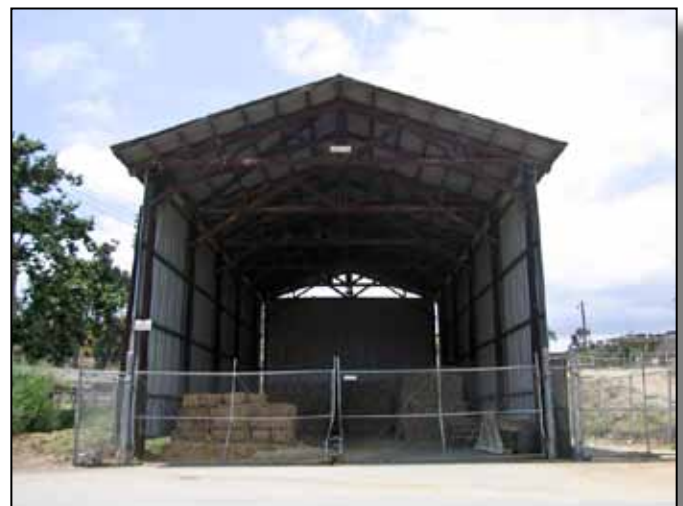
Figure 5.6-9: Current fence conditions at feed shelter. Replace chainlink with Base approved standard fence for this area.
