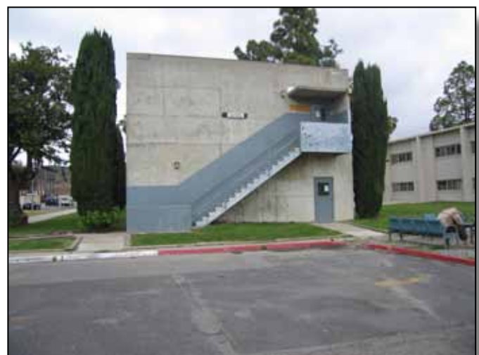
Figure 4.4-10: Rehabilitate existing buildings.
