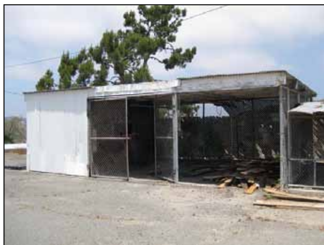
Figure 4.6-6: Abandoned kennels in various states of disrepair atop the knoll.
