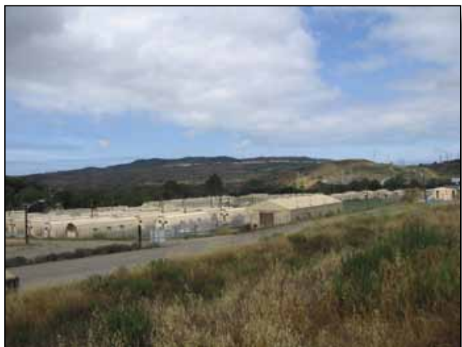
Figure 4.20-4: Quonset huts are the primary structure in the Talega (64) Area.
