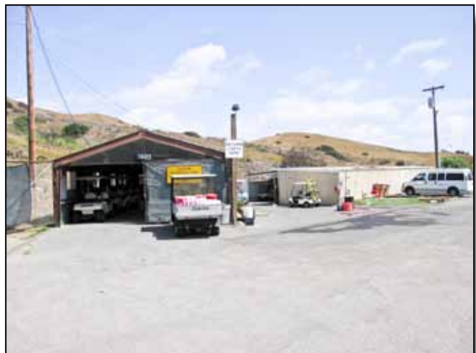
Figure 5.5-4: Maintenance Building 18422 area and storage facility.
