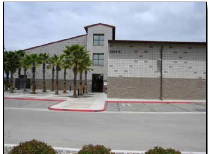
Figure 4.16-12: Existing parking lot that does not meet AT/FP guidelines.
