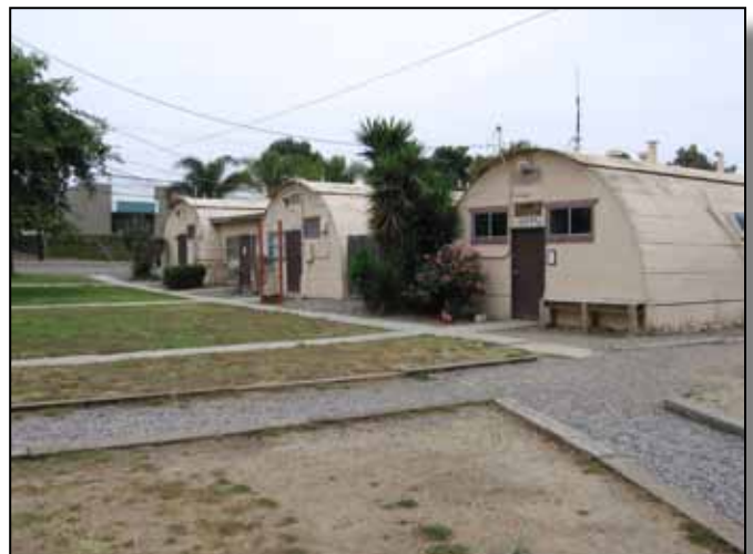
Figure 3.4-3: Quonset huts at San Onofre (52) Area.
