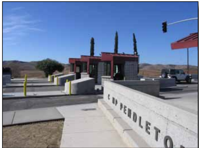
Figure 6.3-2: Sentry stations at San Luis Rey Gate.
