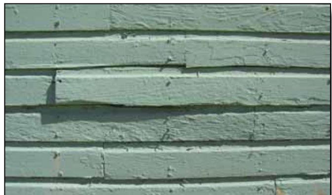
Figure 9.11-1: Mechanized Museum wood exterior.
