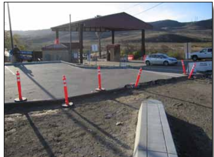
Figure 6.6-4: Vehicle holding area.
